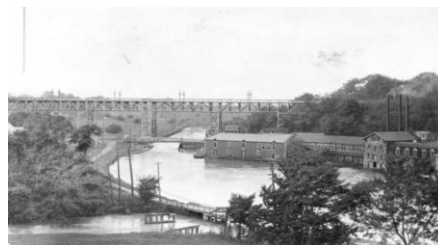
Steel bridge from Glenridge
